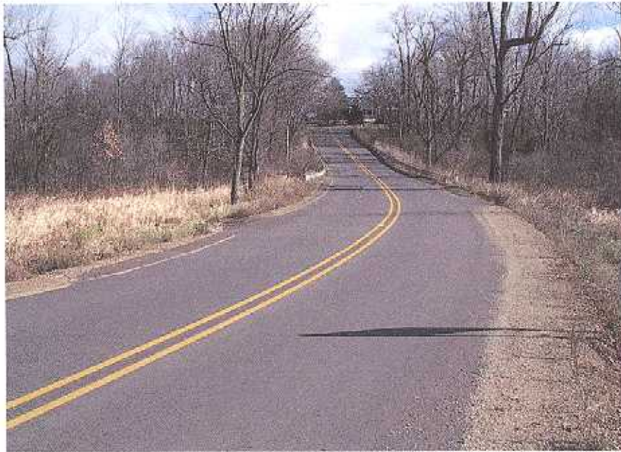
AB AVENUE LOOKING EAST AT FOLLOWING BMP CONSTRUCTION, NOVEMBER 2003
