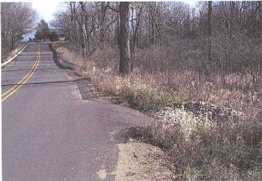
AB AVENUE LOOKING EAST AT SOUTH SPILLWAY, FOLLOWING CONSTRUCTION, NOVEMBER 2003
