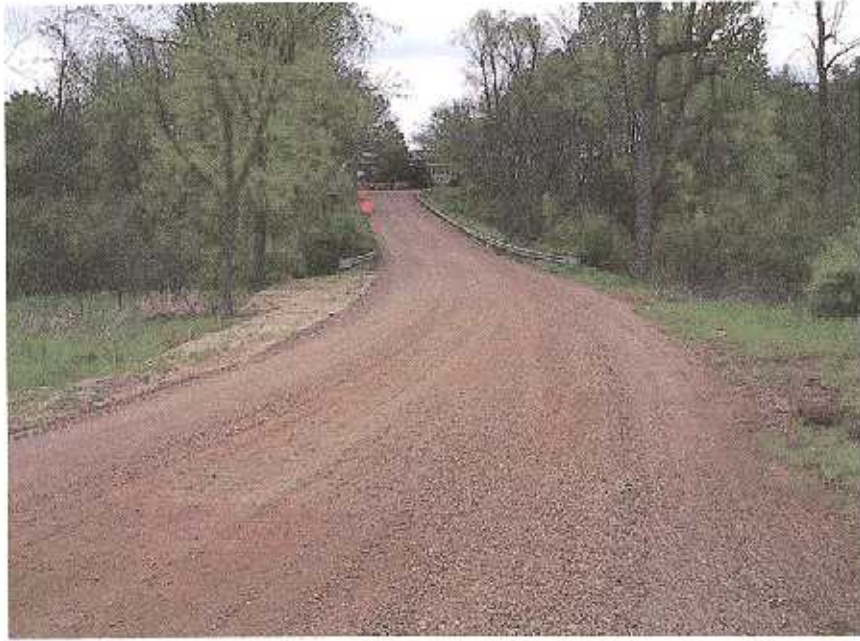
AB AVENUE LOOKING EAST PRIOR TO BMP CONSTRUCTION, JULY 2003
