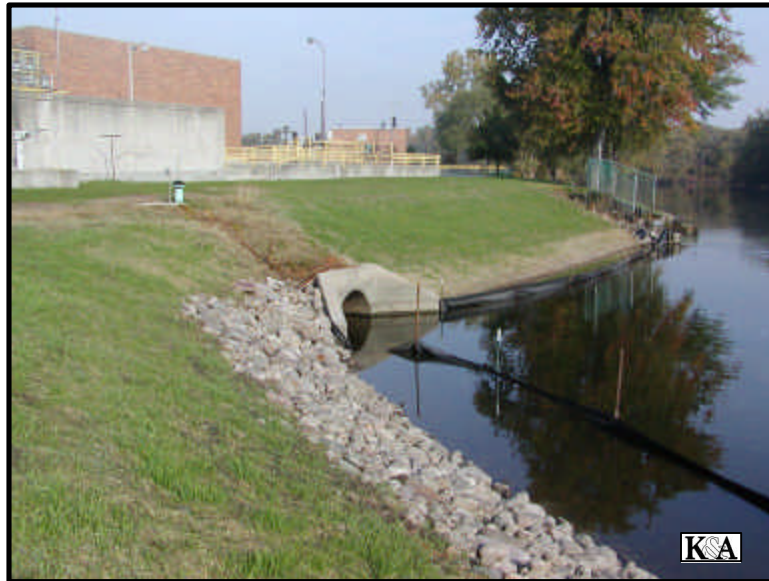
CMI Critical Erosion Site Mitigation Project, Site #10, Kalamazoo Water Reclamation Plant.
