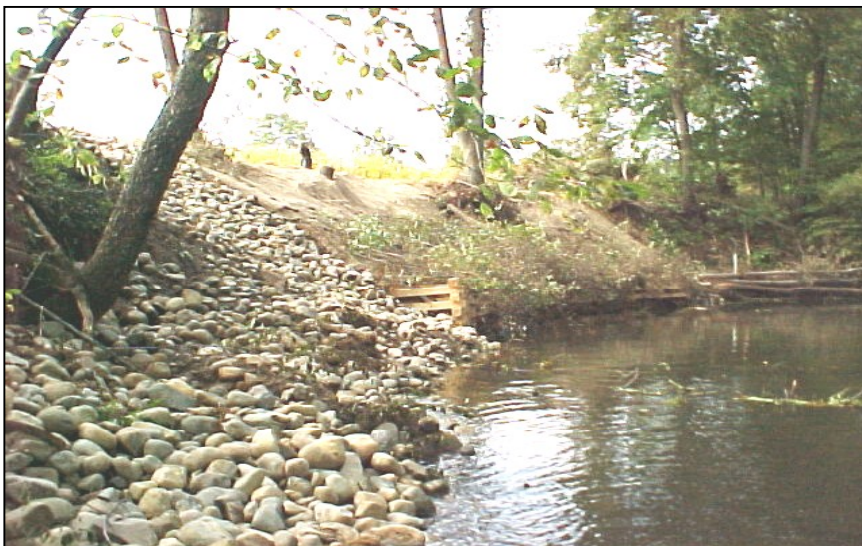
"After" pic showing rock rip rap, crib walls, and vegetation:
