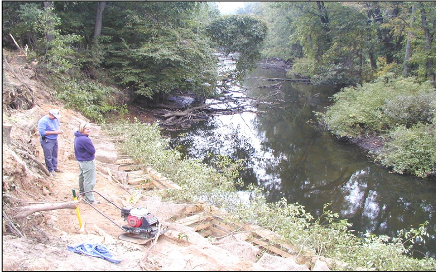
"After" pic showing rock rip rap, crib walls, and vegetation:
