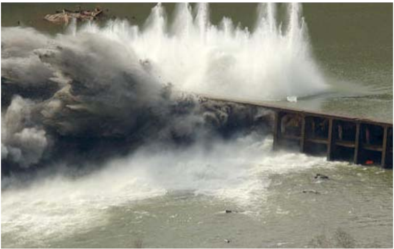
Removal of the Embrey Dam – AP Photograph
